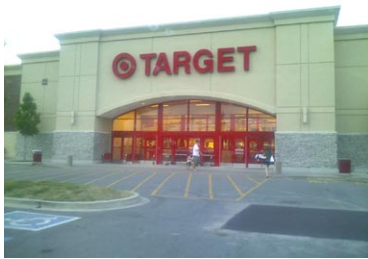
Figure 22.2 (left) This building has been constructed with an easily identified base and cap.
